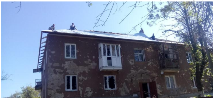
88 households in Semenivka in neighborhood of Slovyansk received reinforced tarpaulin from UNHCR for fast roofing repairs
